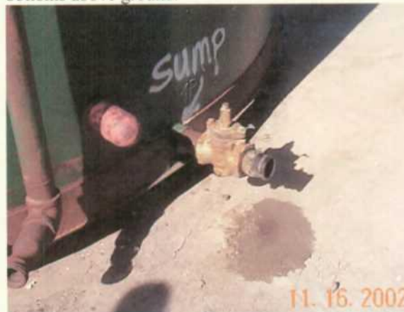
Photo 6. One of the storage tanks had a leaking valve without catch barrel.
