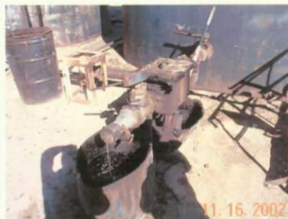
Photo 21. Valve catchments below valves.
