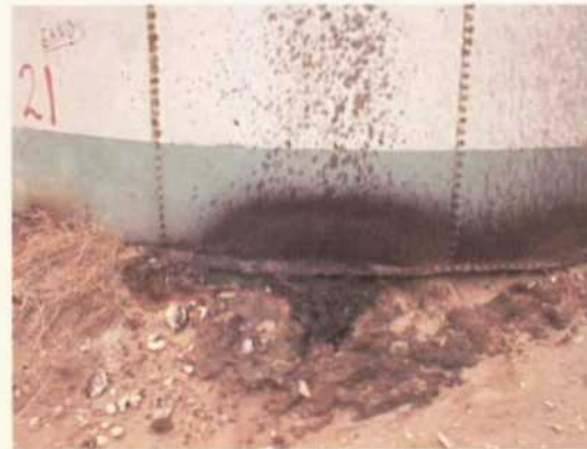
Photo 5 04-11-00 Leaking tank to be cleaned and removed.
