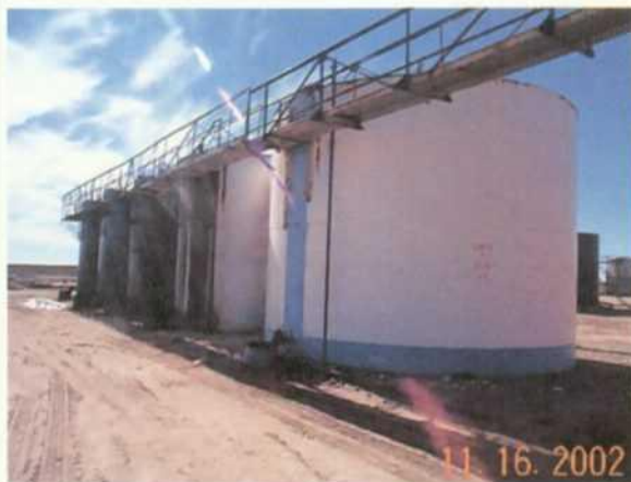
Photo 14. Five oil sales tanks, four 300bbl and one 1000bbl. Catchments were in place and empty.
