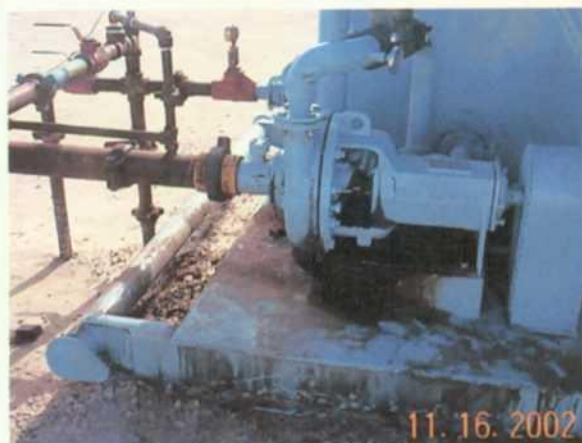
Photo 2. Heating unit pump leaking.
