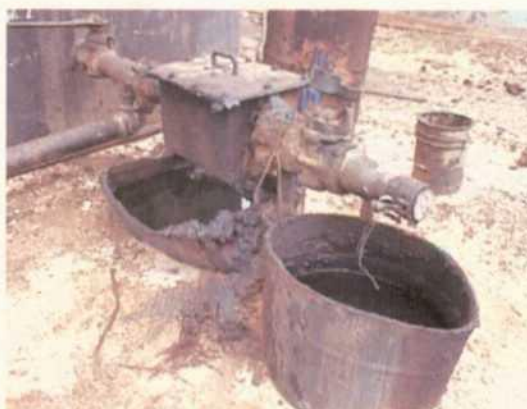
Photo 11 04-11-00 Leaking valve and sumps with oil and water.
