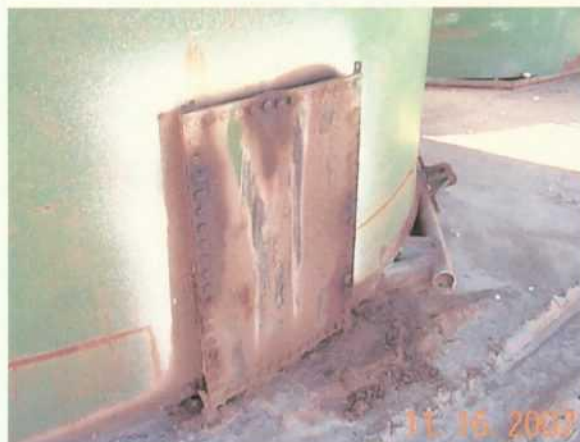
Photo 8. Another hatchway shows evidence of leaking.
