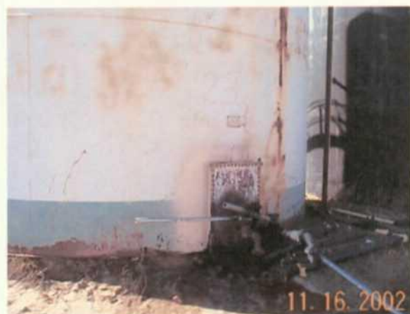
Photo 20. Tank with bottom edge exposed.
