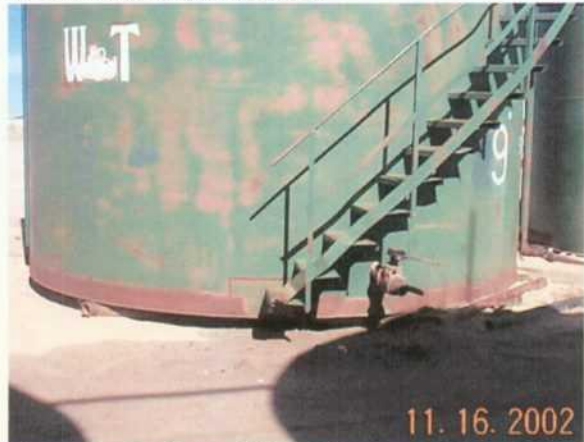
Photo 10. Tanks on skids with bottoms above the ground surface.
