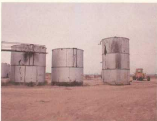
Photo 8 04-11-00 Bolted tanks to be cleaned and removed
