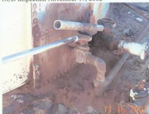
Photo 19. Soil stained with from leaks and spills.
