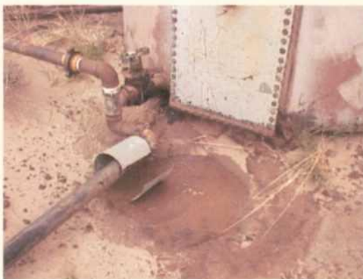
Photo 14 04-11-00 Leaking valve or pipe
