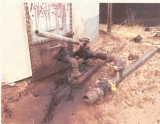
Photo 12 04-11-00 Leaking valve or pipe.
