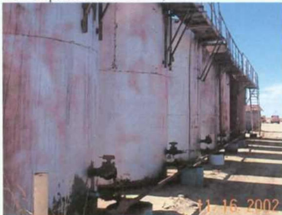
Photo 13. Seven tanks with valve catchments all in place and all empty.
