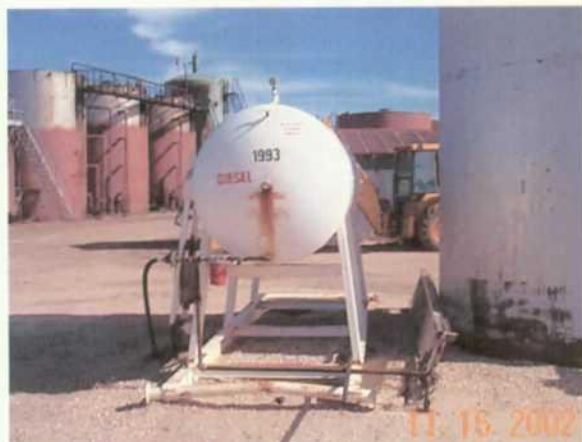
Photo 3. Labeled diesel saddle tank.
