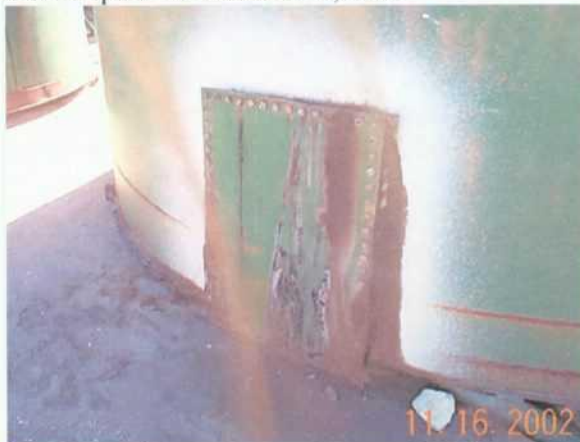
Photo 7. Hatchway shows evidence of leaking.
