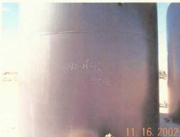
Photo 15. Oil sales tank with Section, Township and Range noted on the side along with the volume.
