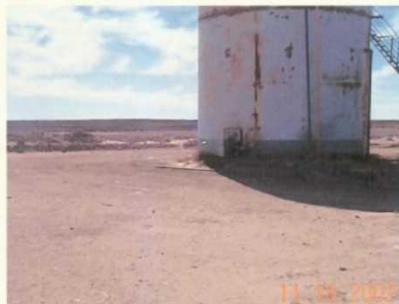
Photo 18. Tank with bottom edge exposed.
