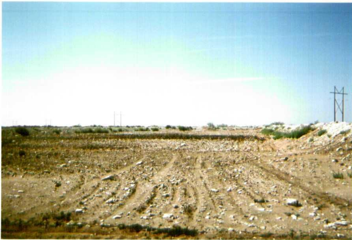
PHOTO 13: Item #2 (Land Farms Operations): The contaminated soil has been spread at the surface to less than six inches.
