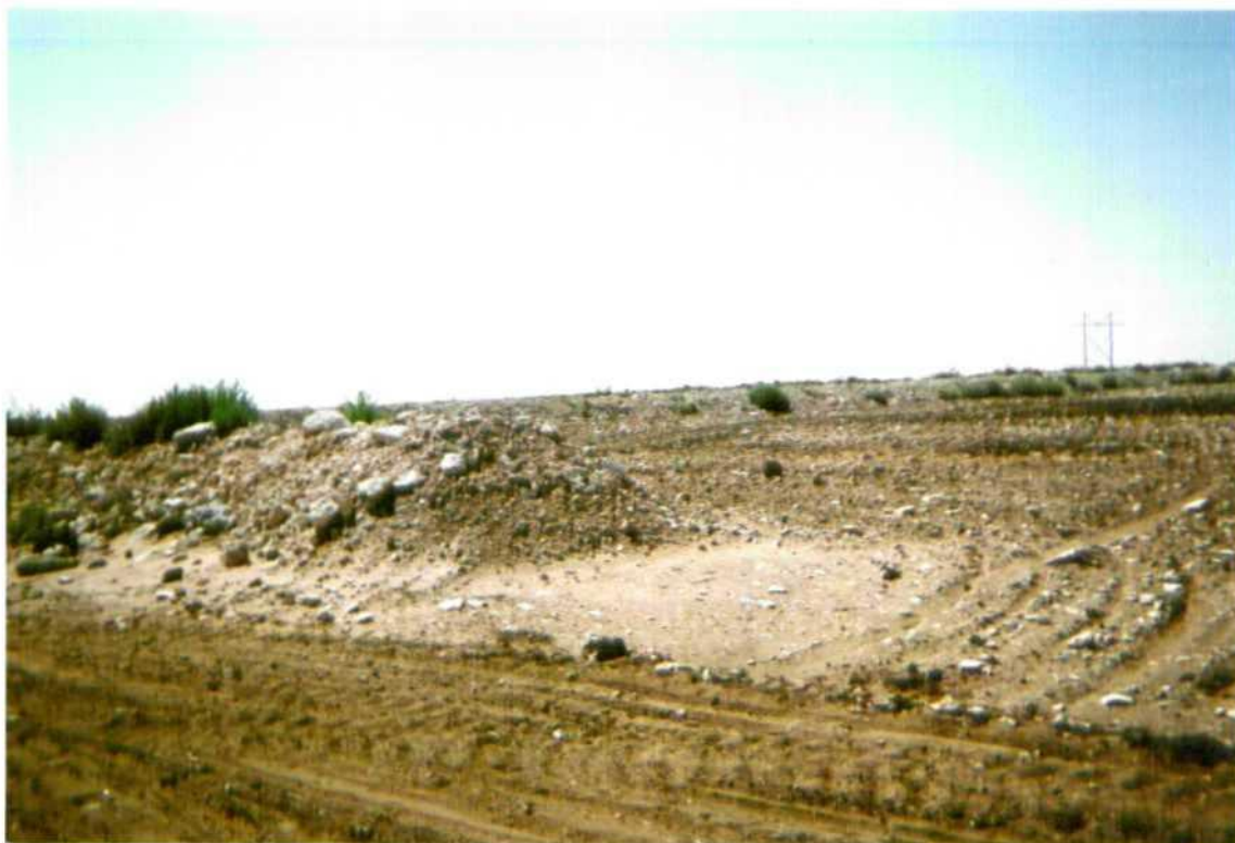
PHOTO 12: Item #2 (Land Farms Operations): The contaminated soil has been spread at the surface to less than six inches
