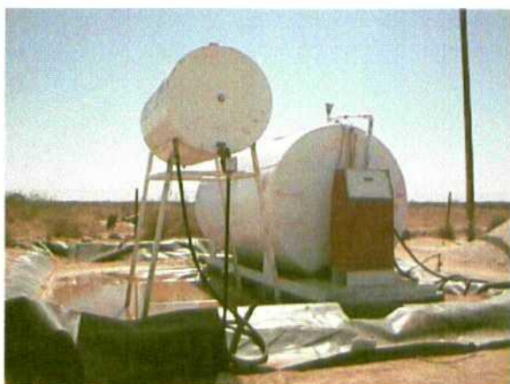
Photo 20 04-13-00 facing east Fuel tank lined containment.
