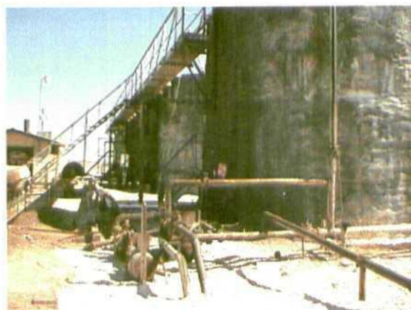
Photo 10 04-13-00 facing north Oil soaked soil covered over and bleeding through.
