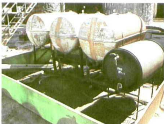
Photo 3 04-13-00 facing east Secondary containment for saddle tanks.
