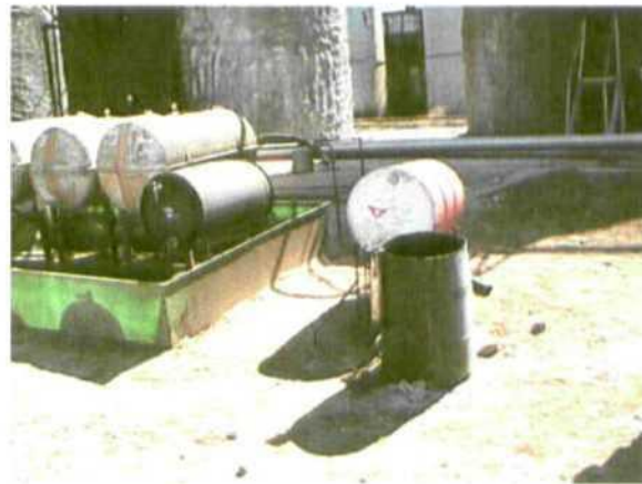
Photo 4 04-13-00 facing east Secondary containment for saddle tanks.
