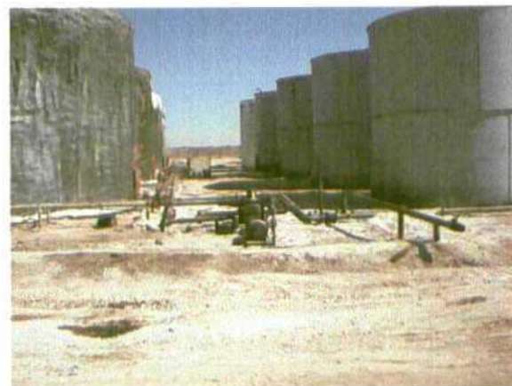
Photo 11 04-13-00 facing north Valves without catchments and oil stained soils.
