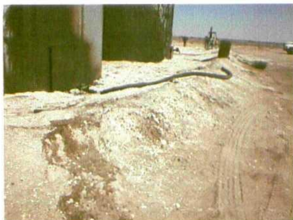
Photo 13 04-13-00 facing north Hose draining directly to ground.
