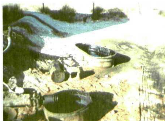
Photo 26 01-20-00 facing west Full sumps and oil contaminated soils from spills.
