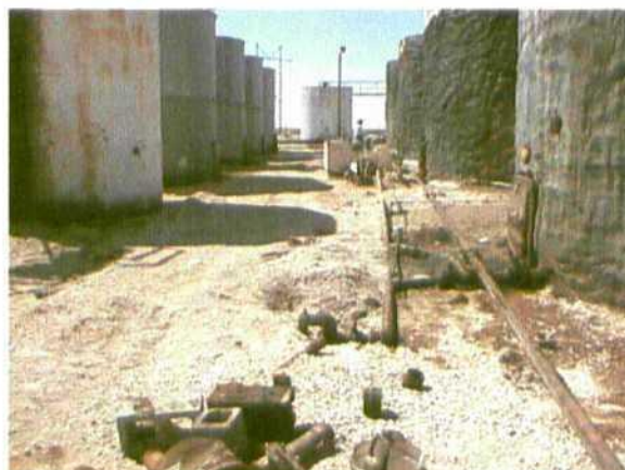
Photo 22 04-13-00 facing south Oil stained soil from leaks and spills.
