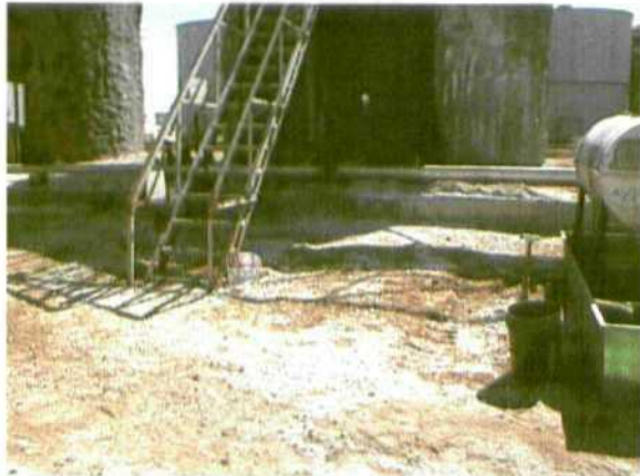
Photo 2 04-13-00 facing east Oil soaked soil covered over and bleeding through.
