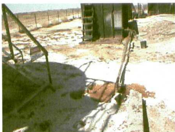
Photo 7 04-13-00 facing west Oil saturated soil from paraffin tank spills and line leak.
