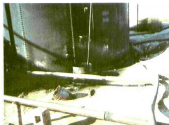
Photo 25 01-20-00 facing west Leaks, spills and full sump.
