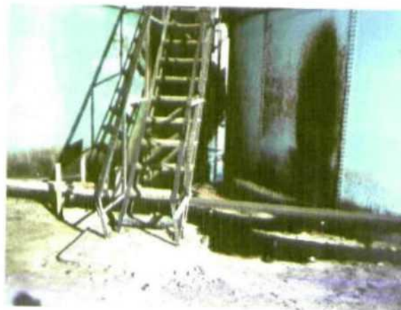
Photo 14 01-20-00 Spills, leaks and standing oil between tanks
