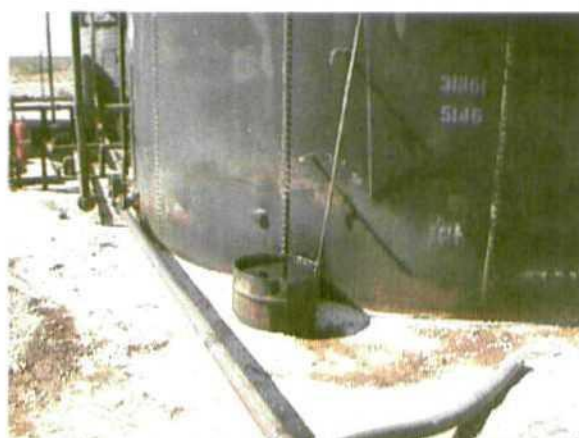
Photo 6 04-13-00 facing south Oil soaked soil covered over and full sump.
