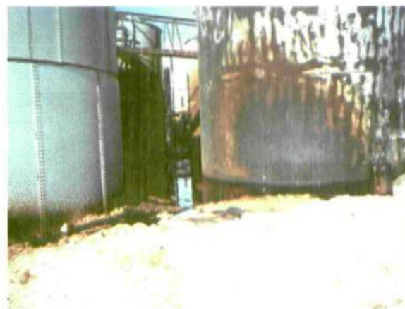
Photo 21 01-20-00 facing west Standing oil back of tanks
