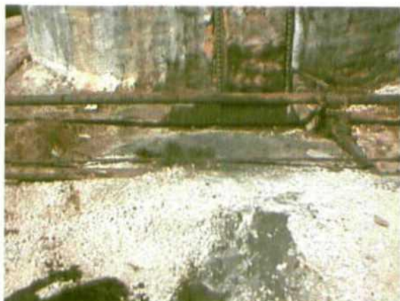
Photo 25 04-13-00 facing west Leaking tank, oil soaked ground covered by clean soil
