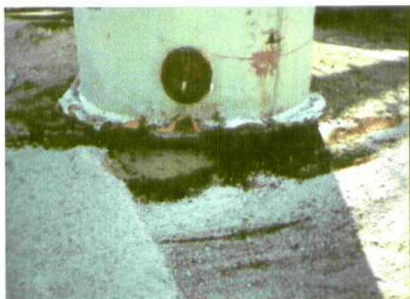
Photo 23 01-20-00 Leaking tank, spills covered with clean soil.
