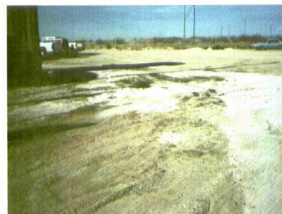
Photo 28 01-20-00 facing west Oil spill that ran down road covered with fresh caliche.
