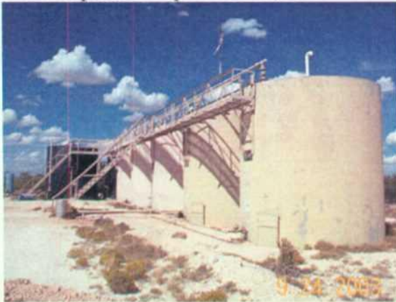
Photo 7. Berm around tanks is low.
