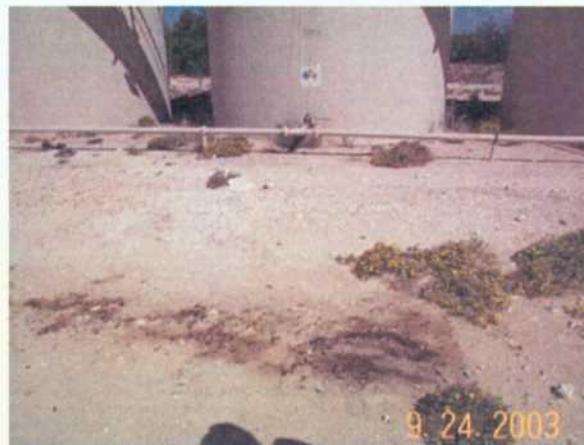
Photo 4. Oil stained soil in foreground. Berm around tanks is very low, less than 1 foot high.
