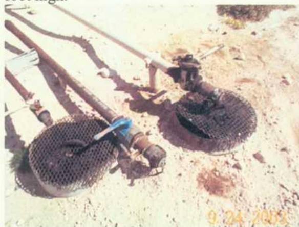
Photo 5. Valve sumps need to be emptied to prevent potential overflows.
