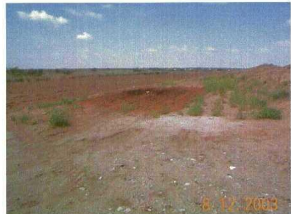
Photo 3: South part of Cell 1. Tilling performed; lift thickness looks to be no more than 6 inches within permit limits. Clean soil pile along right side of photo. Looking west.
