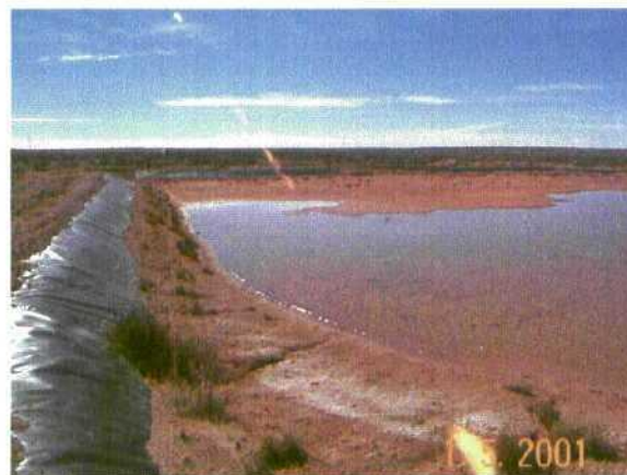
Lined storm water collection pond looking north. Contains snow, rain water and clean soil to hold the liner in place. Propose to use for both facilities.
