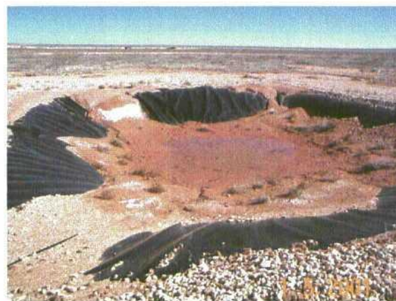
Leachate Collection Pond for the NMED Landfill. Contains snow, rain water and clean soil to hold the liner in place.
