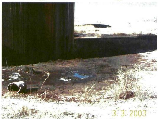
Photo 7: Contaminated soil surrounding the leaking 500 bbl tank.
