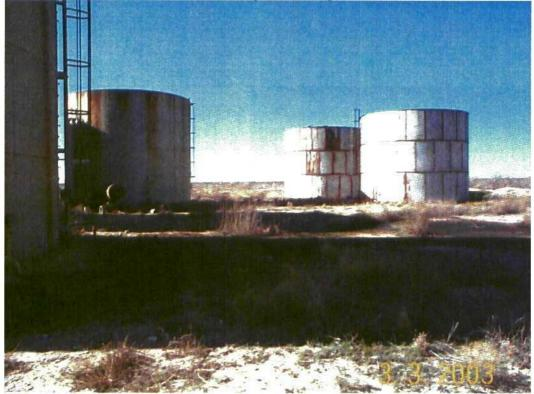
Photo 8: Contaminated soils and 4-500 bbl tanks. Looking southwest.
