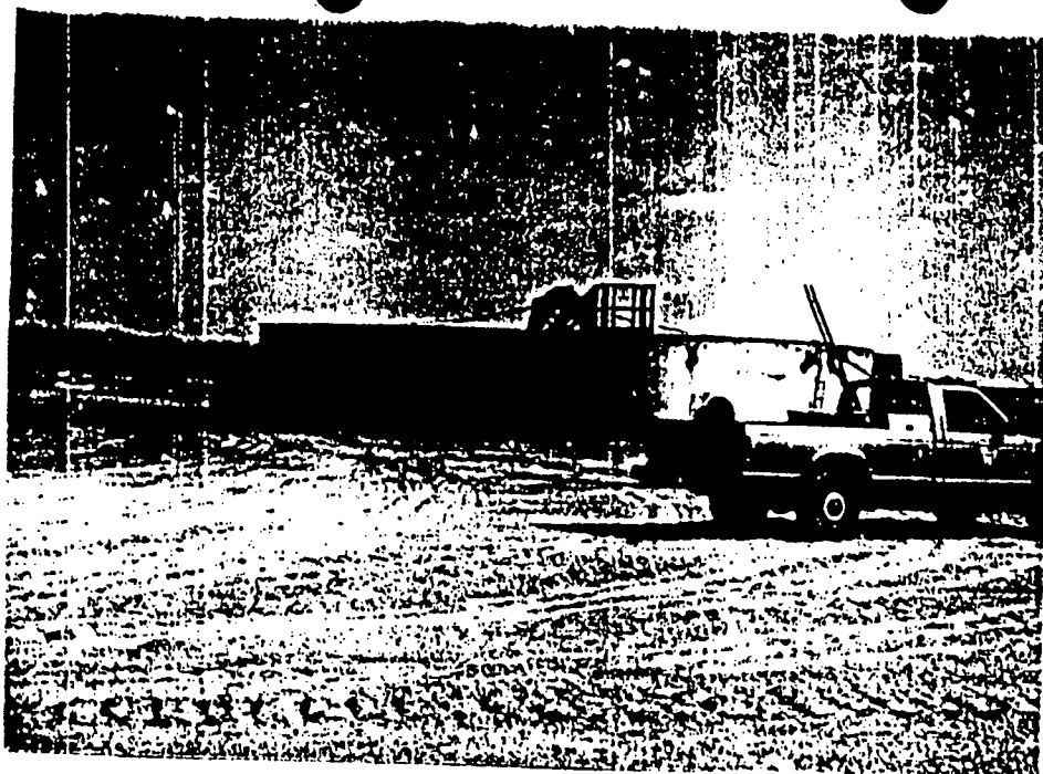
Photo No. 3. Southwest view of the aeration unit of the B & E Trucking salt water disposal facility located adjacent to Laguna Qatro. Note the produced water at this unit is processed through a series of separation tanks, not shown, prior to entering the aeration unit.
