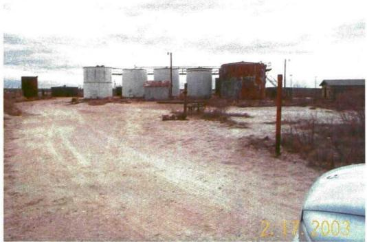
Photo 12. From left to right, 1-210 bbl welded tank, 1-250 bbl bolted tank, 1-500 bbl bolted tank, 3-500 bbl welded tanks, 10'x10'shed, 2-750 foam insulated tanks, enclosed LACT unit and 2'x30' shed. Looking east.
