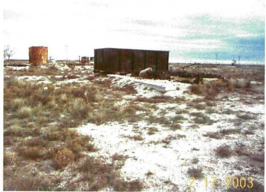
Photo 3. 36x20 concrete pad with dried paraffin piles on pad. Steel plate box 8'h x 20'w x 10'l set on north end of concrete. Looking north-northeast
