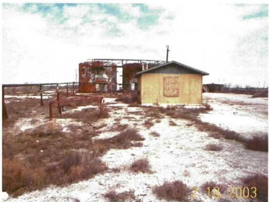
Photo 10. From left to right, 2-750 bbl foam coated tanks, 20'x 30' office building and 1-250 bolted tank. Looking North.
