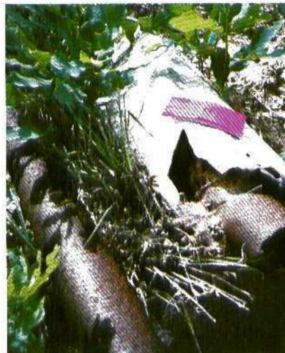
Sample 17: Insulation north small on-ground pipe run
