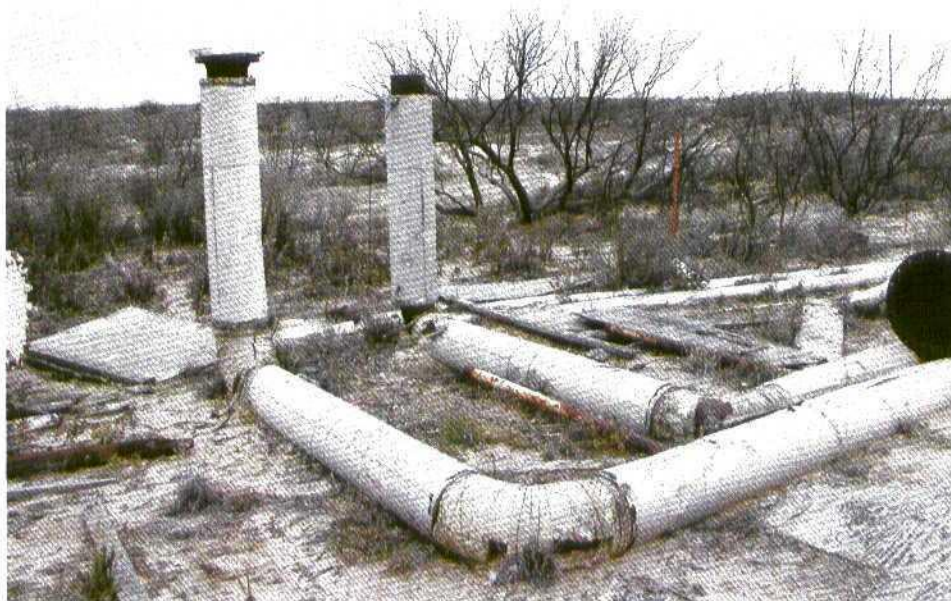
Photograph No. 1. Asbestos-coated piping located north of the lease road. All piping and asbestos were disposed of during site reclamation.
