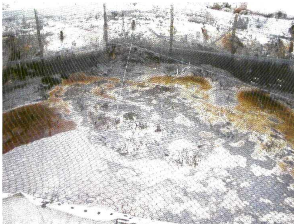
Photograph No. 3. A 1,200-barrel buried tank filled with oil field waste. The tank was located south of the lease road, which was cleaned, excavated, and disposed of during the site reclamation.
