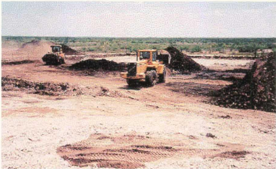
Construction of biopiles at the Goodwin Treating Plant site.
