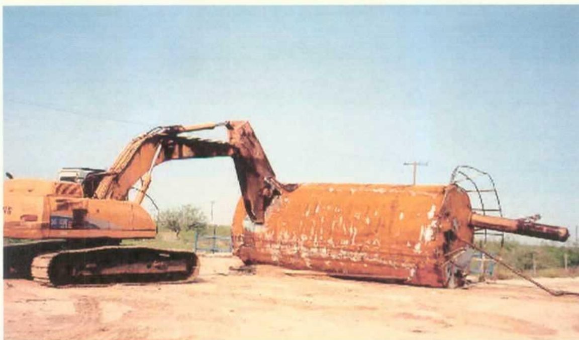
View of Treater being dismantled.
