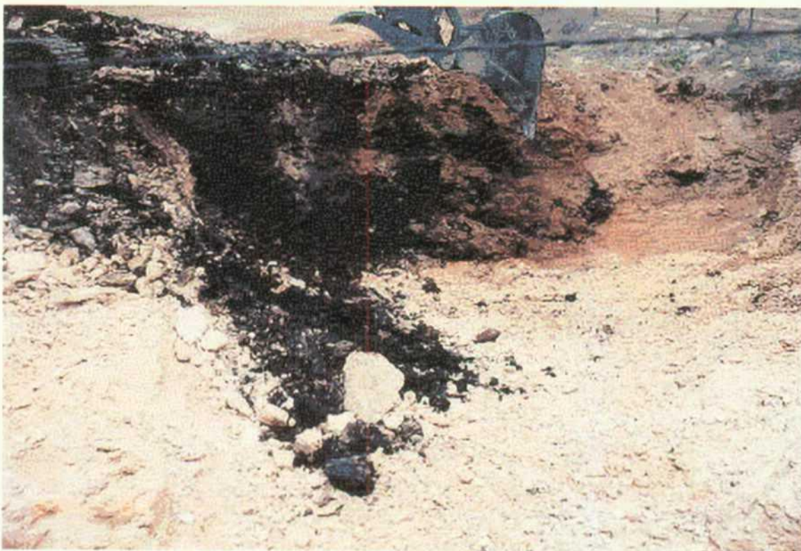
View of hydrocarbon-impacted soils excavated from the Goodwin Treating Plant site.
