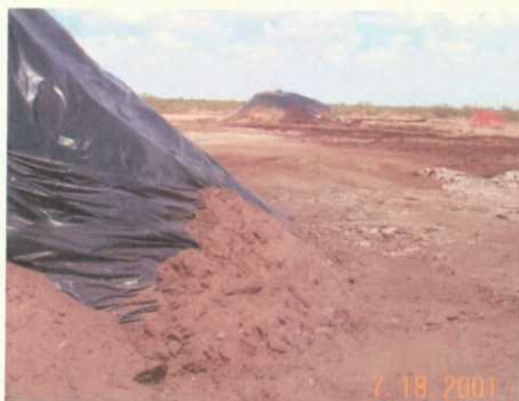
Contaminated soil piles and tank foot print areas.
