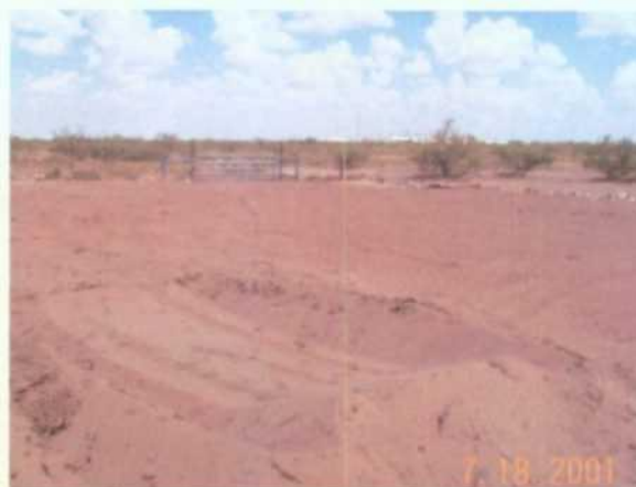
Overflow pit back filled with clean soil.
