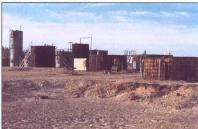
The soil boring/monitoring well will be located in the overflow pit located on the southeast corner of the site (foreground in the photograph)
