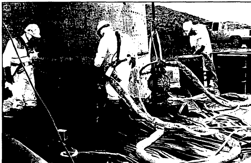
Tank and vessel decontamination
