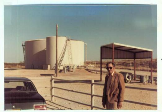
10,000 Bbl. Effluent + Water Storage Tank and 750 Bbl. Brive Water Mixing Tank
