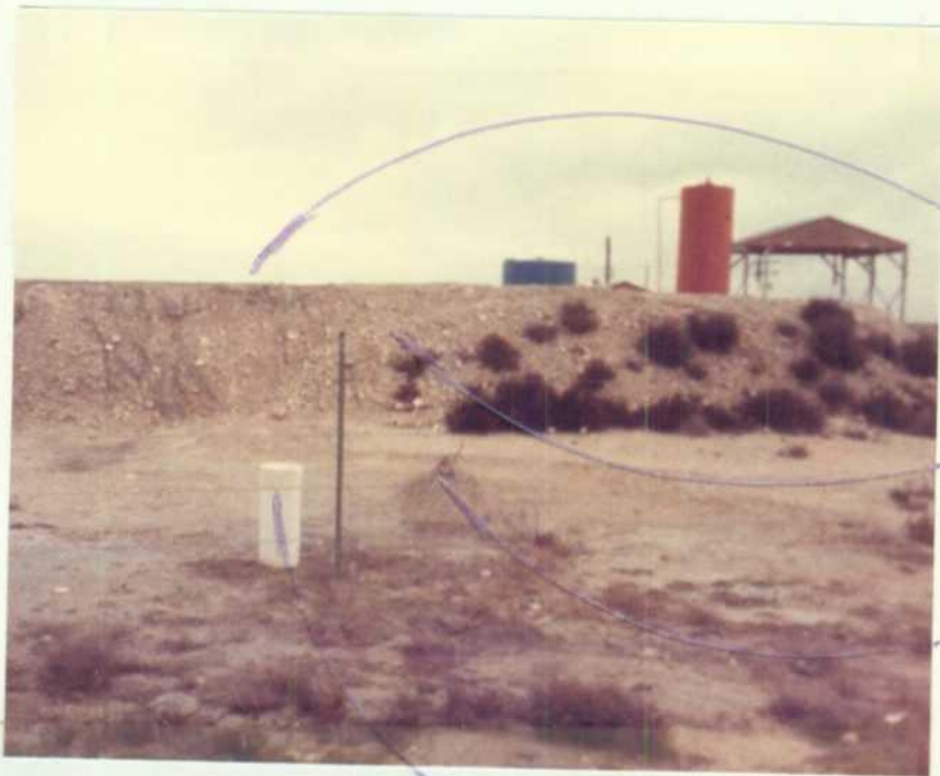
SEEPAGE INSPECTION PIPE
