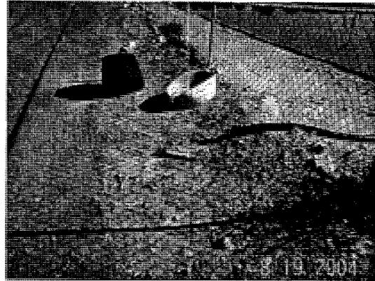
Loading area west of Brine Pond. Visual salt contamination on ground. No containment devices.
