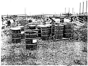
Drum storage area with "Selectox TM 33" on S side of plant violates drum secondary storage provisions of permit. No impermeable pad with curbing was present and empty drums are not stored on their sides (8-17-06)
