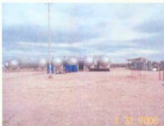
Bullet tanks- some these tank currently hold liquids other than propane/butane- No secondary containment observed.
