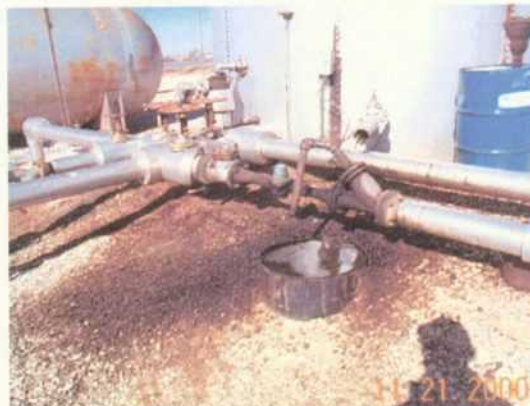
Pic#5- Class II SWD disposal well area filter screen drain sump.
