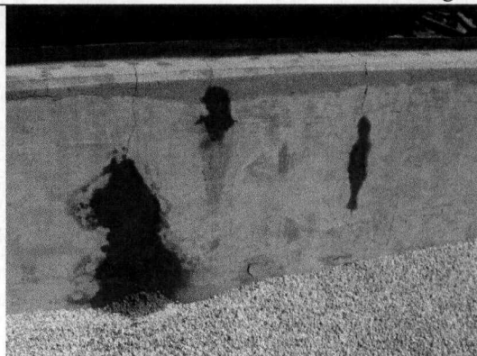
Photo 16: Integrity of compressor skid with cracks.
