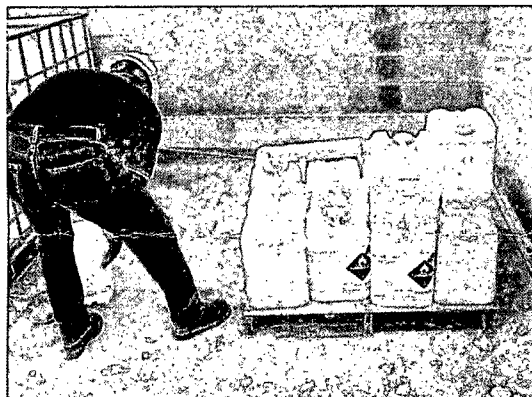
Photo 3: Empty container storage area without proper containment.
