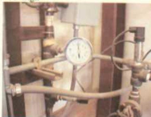
#11 Annulus Pressure gage & high-limit control device.
