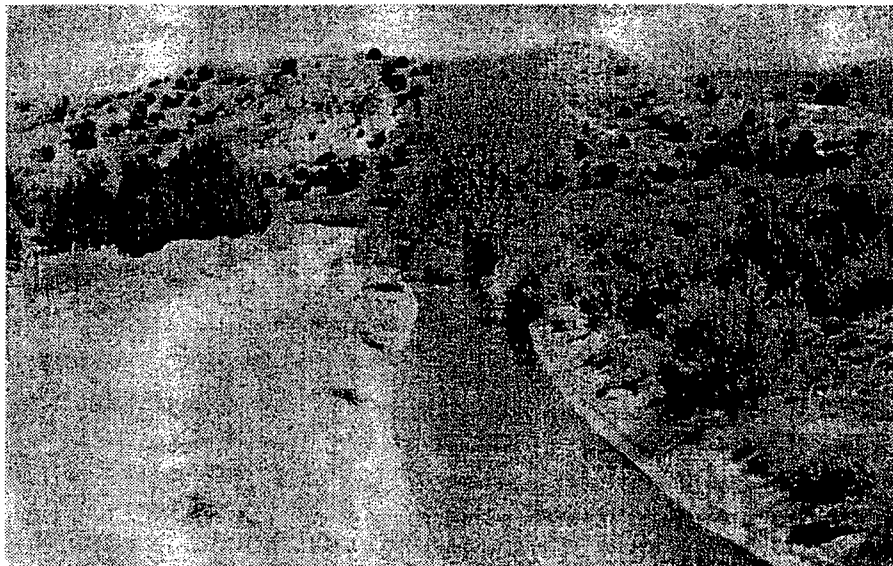
Existing lined section in foreground, unlined in background.
