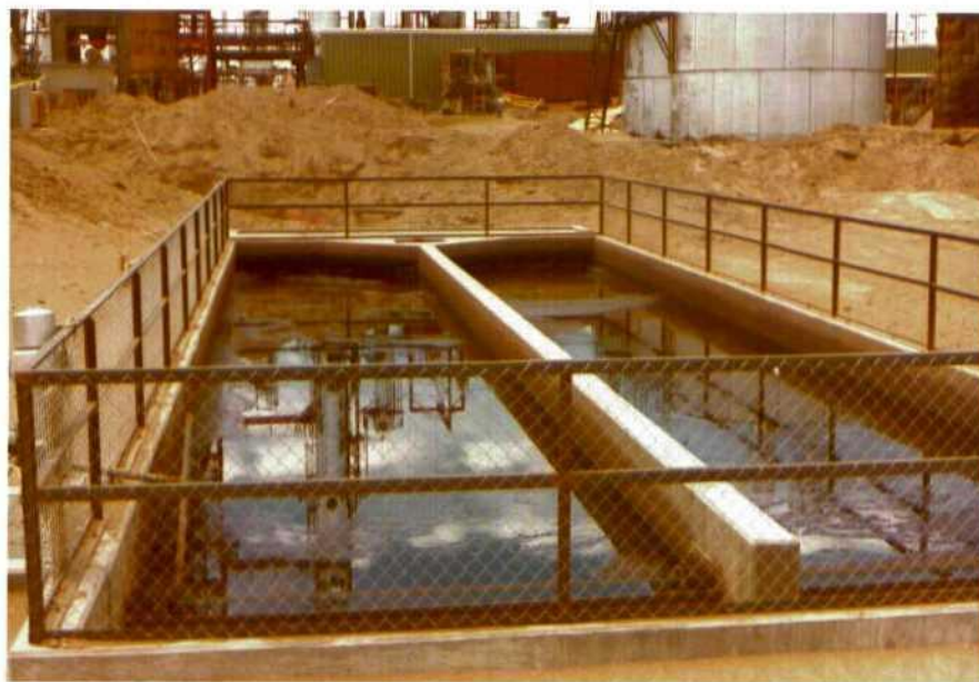
Figure 16. API separator at the Plateau refinery.
