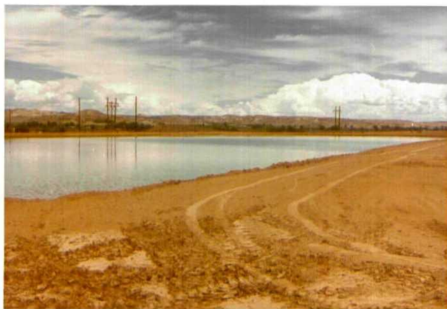
Figure 6. View of solar evaporation pond #1, taken shortly after the pond was filled with fresh water. The silt of the Jackson Lake Terrace forms the pond embankments.
