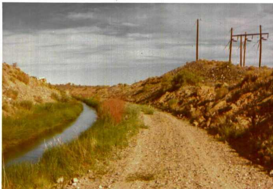
Figure 8. View of the Hammond ditch immediately north of solar evaporation pond #1. Note that the spoil piles on the right hand side of the ditch are primarily comprised of cobble. The spoil piles rest above undisturbed silt.
