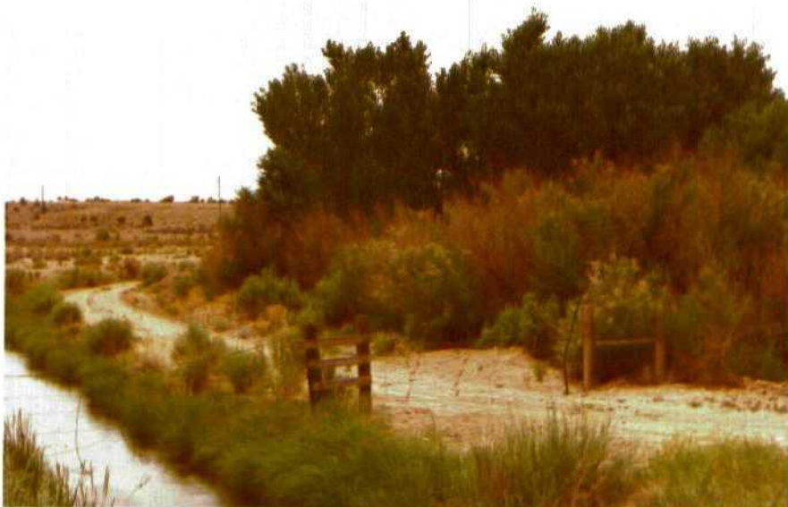
Figure 9. View of the Hammond ditch immediately west of the Plateau Refinery. The dense vegetation to the right of the ditch is supported by leakage from the ditch.
