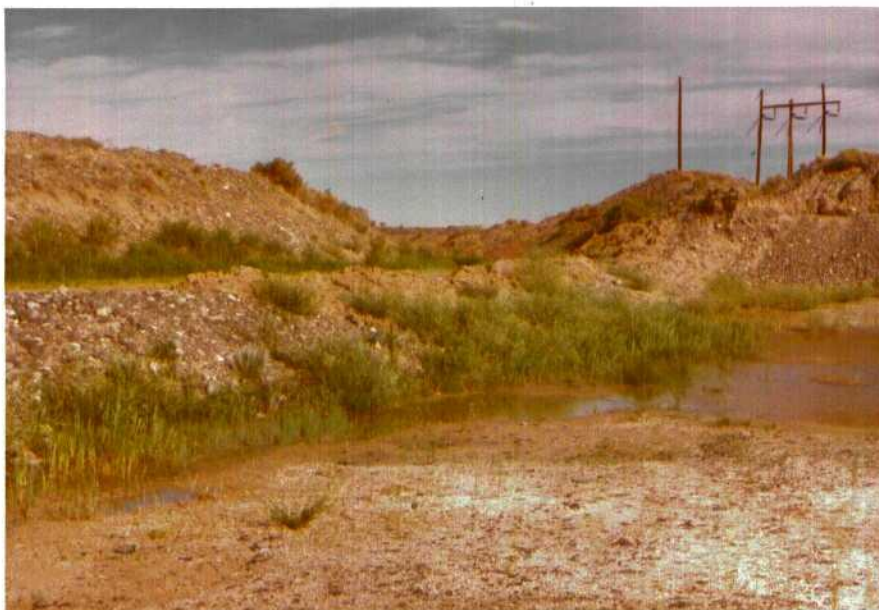
Figure 10. View to the west immediately north of solar evaporation pond #1 showing leakage from the Hammond ditch. The ditch runs from left to right through the photograph but is hidden by the spoil pile on its right bank. Note the cobble in the spoil pile.
