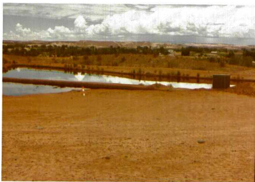
Figure 17. View to the south showing the two oily water ponds at the Plateau Refinery. Pond #1 is in the foreground and pond #2 is in the background. Note the silty soil in the foreground and forming the embankments of the pond.
