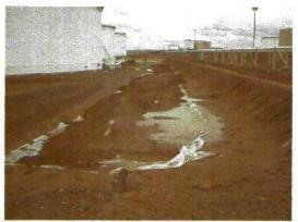
Pic25- Tank 11-14 picture looking east shows where reformate gasoline contaminated soil is being stored on plastic. Pictures shows rain water from recent rains.
