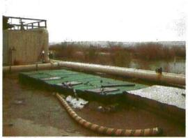
Pic4- Salt Vault used for liquid brine storage to regenerate water softeners. Background shows fresh water duck and geese ponds.
