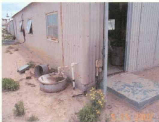
Picture # 3- Product Injection Pump House and waste pump oil sump single wall.
