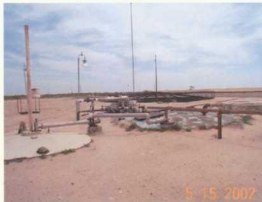
Picture # 5- Out of service Oil/Water separators below grade tanks.
