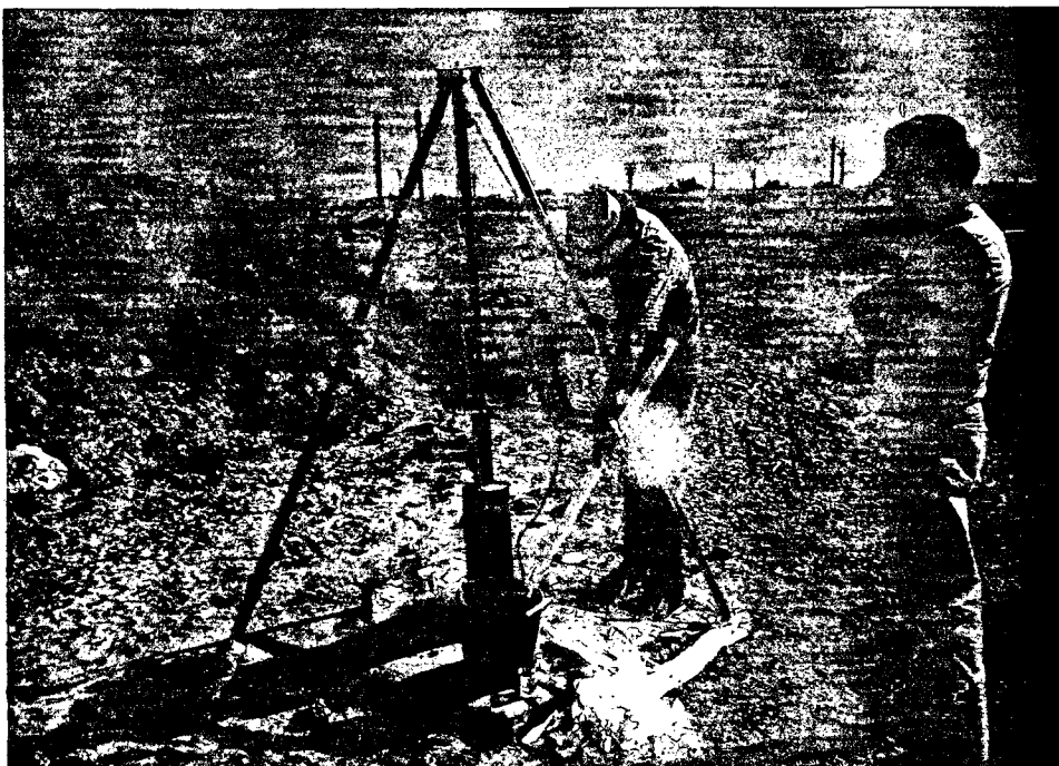
Photo 7: 2:20; 10/26/88; Evacuating MW-3; note Teflon bailer and propylene rope; surface impoundment berm is in left background.
