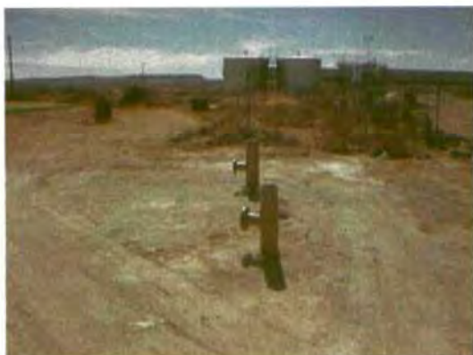
Two new groundwater remediation recovery well.
