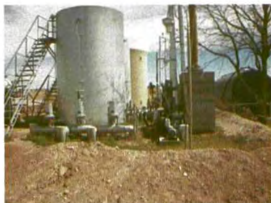
Groundwater remediation treatment system.
