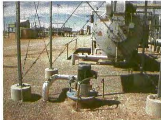
Sump (single containment) for open drain system
