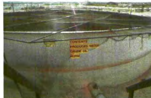
Old water/condensate skimmer basin area tank. Out of service.
