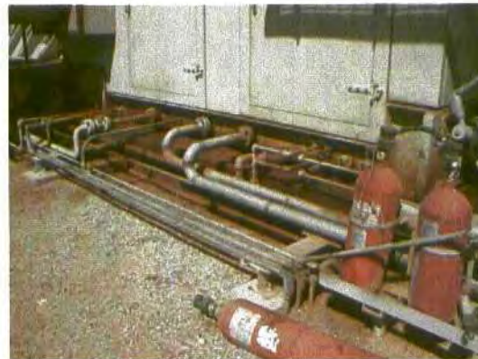
Inlet gas turbine skid.
