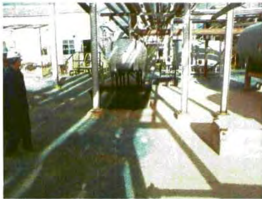
Process area in plant does not have containment.
