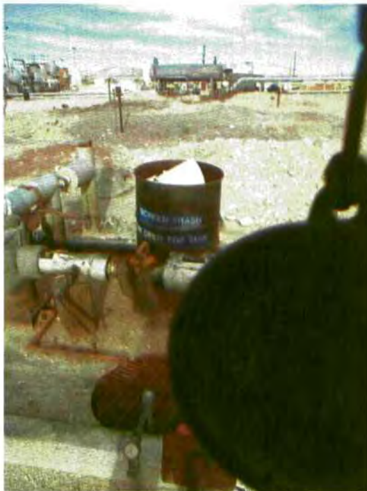
Old Skimmer basin area including out of service pump and sump. Looking east.
