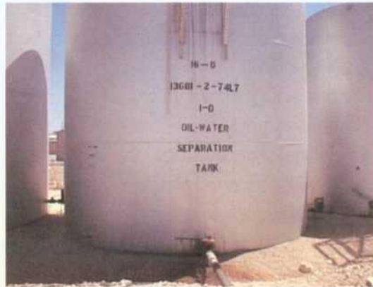
Pic#4 Plant Oil/Water separator tanks.
