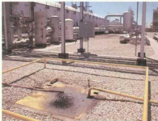
Pic#2 East sump for compressor room. Single wall construction.
