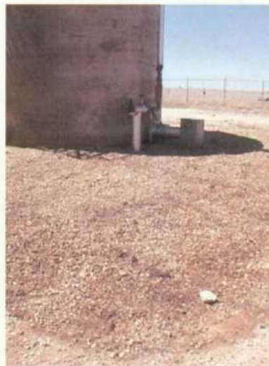
Pic#6 Waste water storage tank- Contaminated soil visible from recent and past releases.
