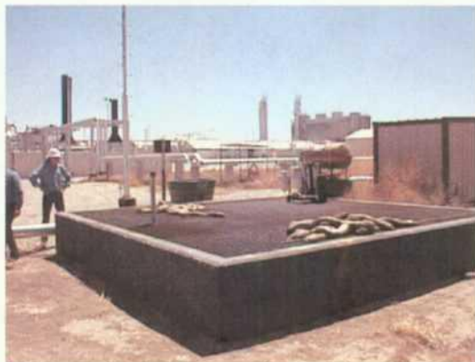
Pic#3 Main Plant Sump with double wall containment.
