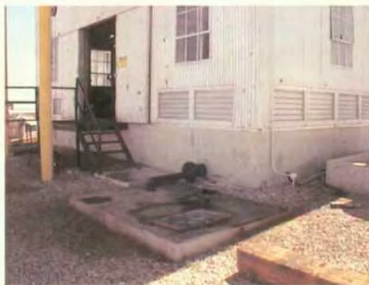
Pic#2 Generator room sump has secondary containment.
