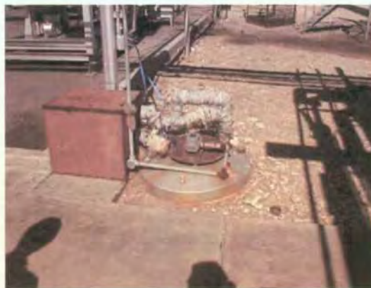
Pic#4 Glycol sump has secondary containment.
