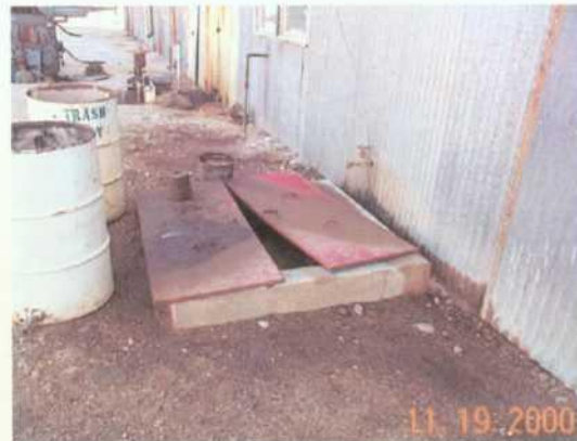
Pic#4- Single wall sump located north of compressor bldg.-
