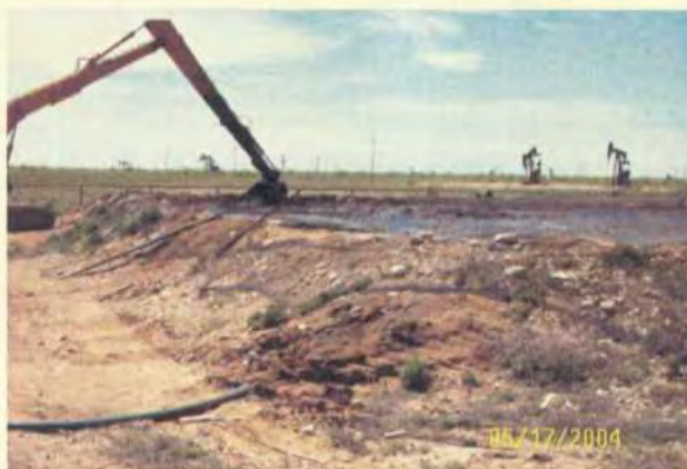
Photo 3. Southwest corner of pit. Pit waste thickness is 4'6" thick. Measurement taken by CRI personnel. Pit appears to be built up on surface.
