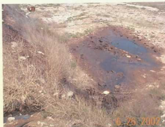
Photo 4: Pit overflow into unlined bermed area approximately 10x11 feet
