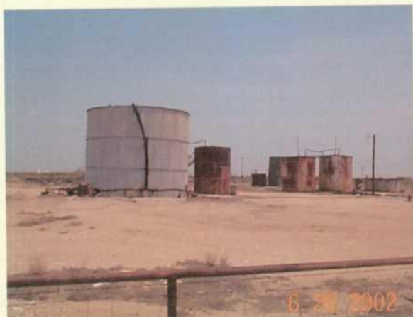
Photo 2: One 3000bbl tank 1/3 full and other assorted tanks. Surface soil very spongy and loose no vegetation. Looking North
