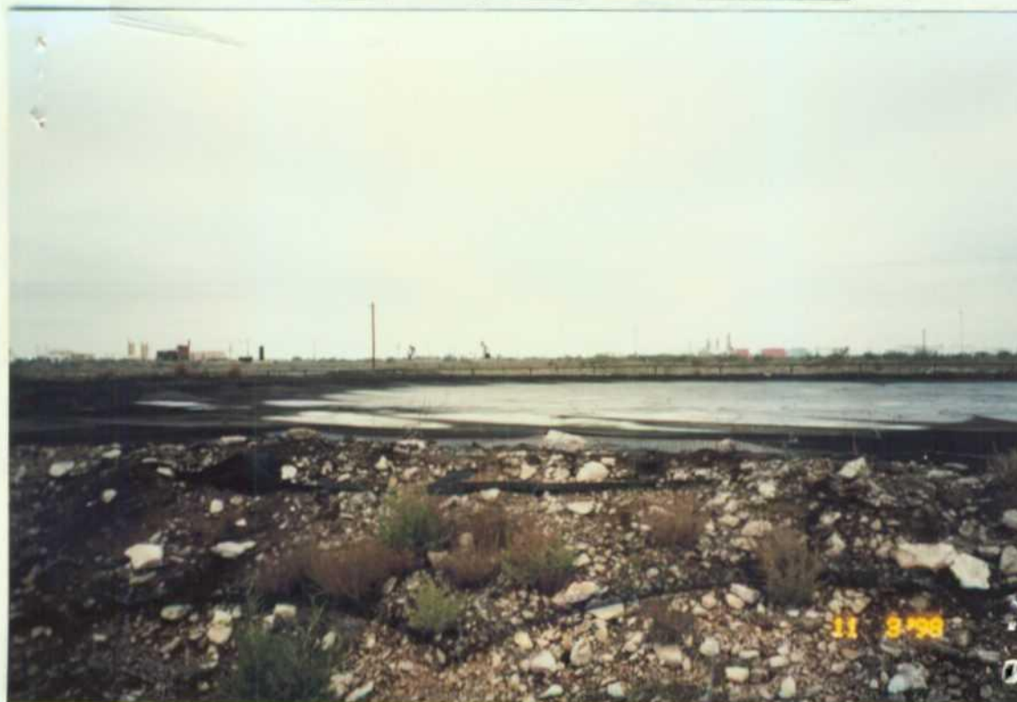
Photo Number: 6 Photographer: T. Reeves, SAIC Location: Araho, Inc. Subject: Pit covered with oil, little freeboard, submerged netting City/County: Lea County State: NM Date: 11/03/98 Time: pm Weather: cloudy
