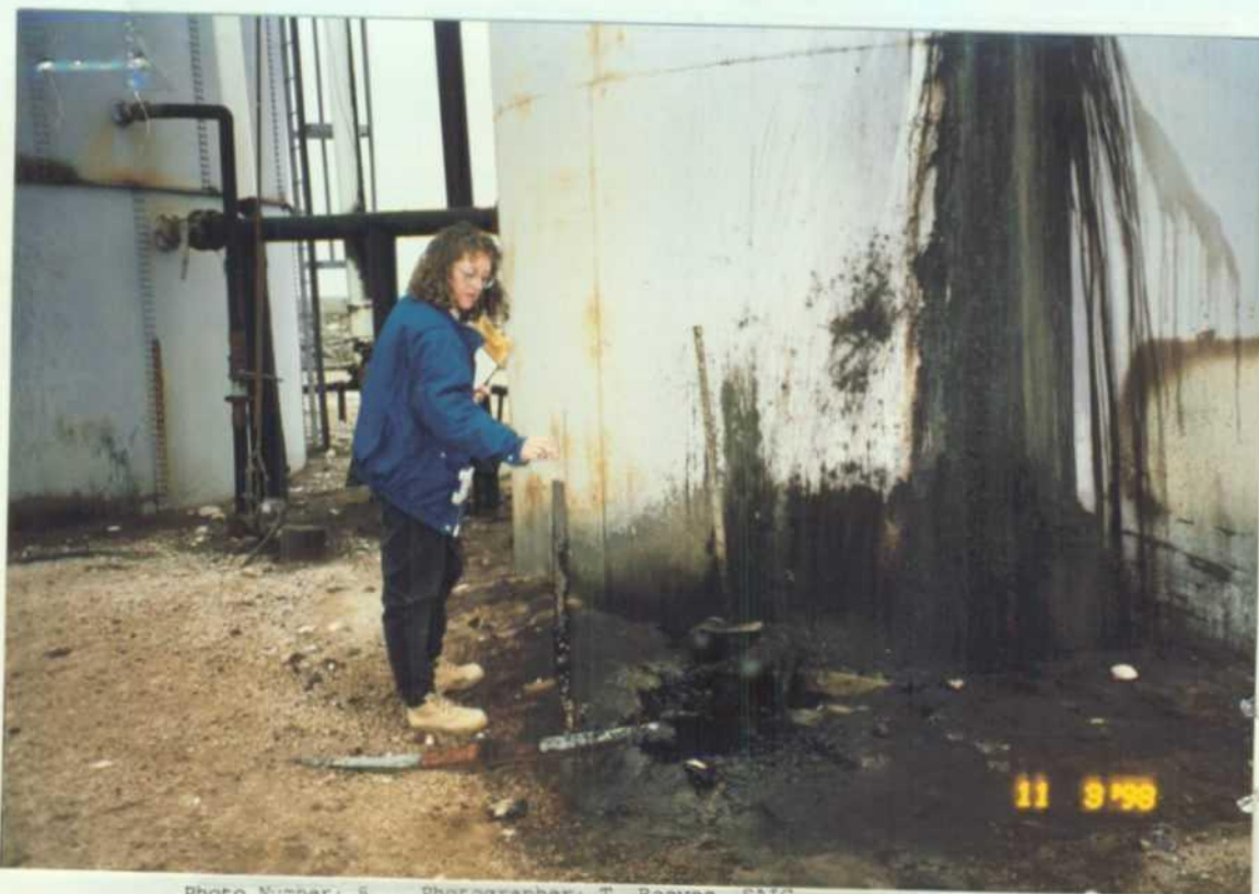
Photo Number: 5 Photographer: T. Reeves, SAIC Location: Araho, Inc. Subject: Sump full of oil beneath tank valve (measured with stick) City/County: Lea County State: NM Date: 11/03/98 Time: pm Weather: cloudy
