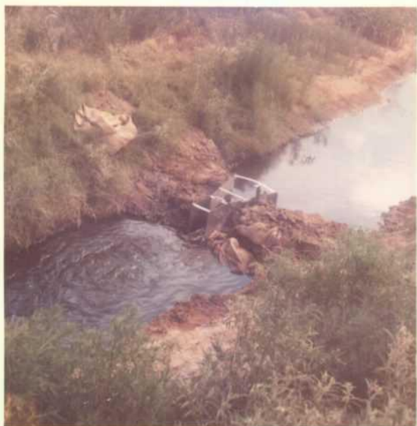
Six-inch Parshall Flume Looking Upstream (Location B)
