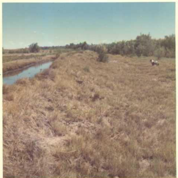
Effluent Ditch Looking Southeast (down- stream) (Ditch is elevated in this area. There was evidence of Ditch overflows here. (Location H)
