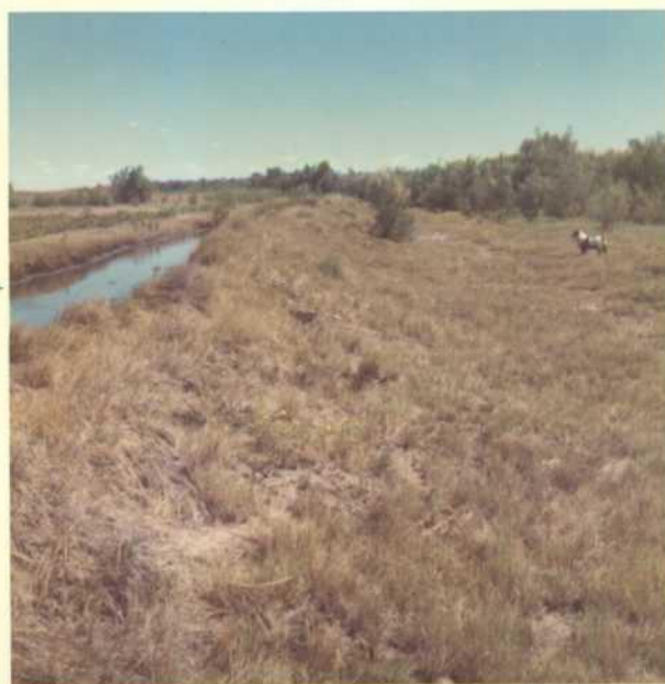
Effluent Ditch Looking Southeast (down- stream) (Ditch is elevated in this area. There was evidence of Ditch overflows here. (Location H)
