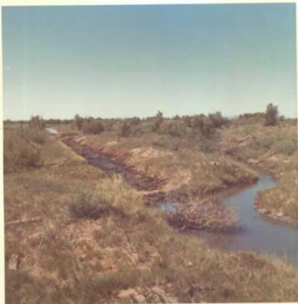
Diversion in Effluent Ditch Looking Northwest (upstream). There was evi- dence of overflows here. (Location K)
