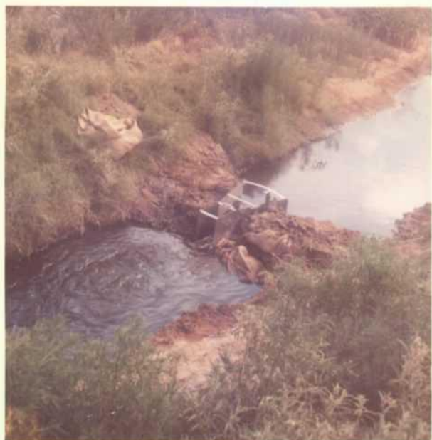
Six-inch Parshall Flume Looking Upstream (Location B)
