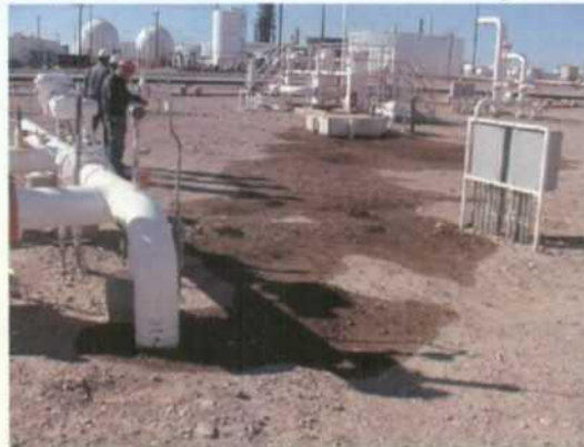
Pic #4- Crude oil pipeline pump area spill. Sump overflowed oil.- Requires action.
