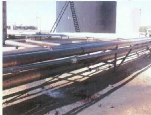
Pic #13- Active leak in CBO line North Plant N Tank Farm. Near LCO and CBO Tanks. Requires action.
