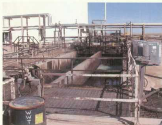
Pic #15- North Plant API Separator. ABT tanks shown in background. This separator is single wall and will be scheduled for inspected.
