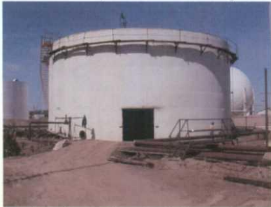
Pic #11- South Plant Tank Farm. Tanks 417, 418, and 419. Area. 418 & 419 Tanks are being repaired. Tank above is receiving new floor and top. One tank 419 (Diesel) in this area was recently repaired and noted to have been leaking. This area requires an investigation to determine contamination extent.
