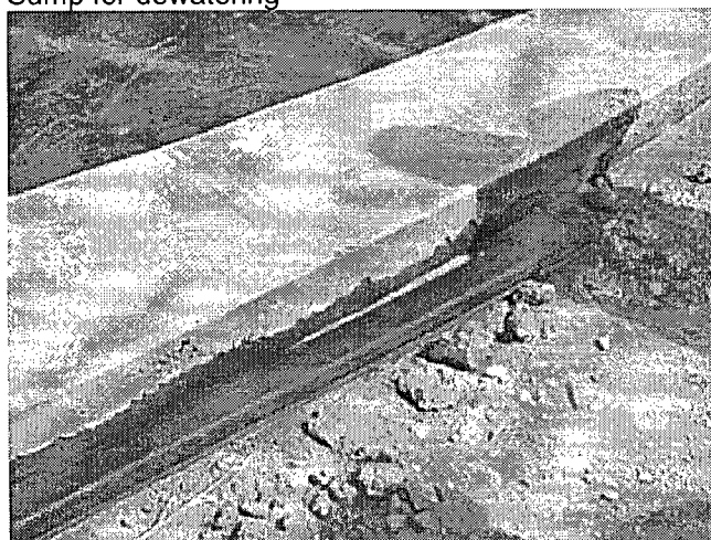
Impermeable liner to be thermally seamed outside of cement ring wall and over and trenched into outer berm area.
