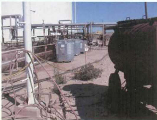
Pic # 16- AST's chemical tote tanks located next to Main API Separator needs containment.
