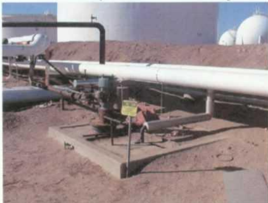
Pic #1- Main blender tank farm sump-single wall.
