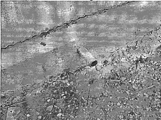
Some older tanks built on cement ring are unlined but have 1 inch PVC pipes set beneath tanks
