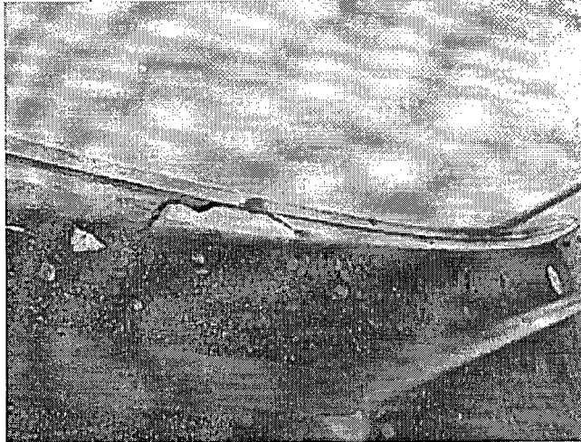
Concrete fracture(s) every 20-30 feet along the circumference and base of the tank.
