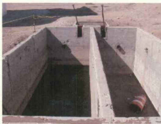
Pic #10- Old API separator located near the south side asphalt tank farm. Requires closure. Standing fluids.
