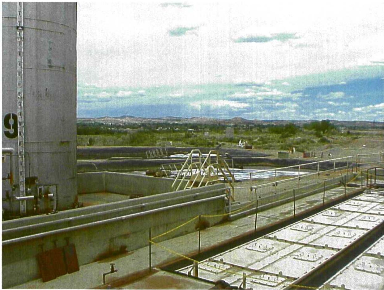
Photo 8 API separator (foreground) and aeration lagoons (background), facing northeast
