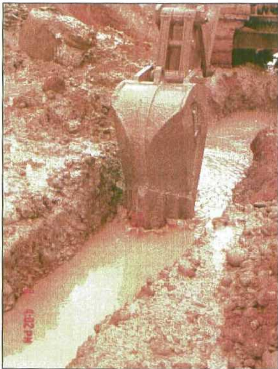
Rock bucket used to excavate through the Nacimiento Formation.
