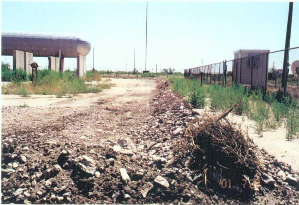
5. Storm Water Retention Berm (Looking East)
