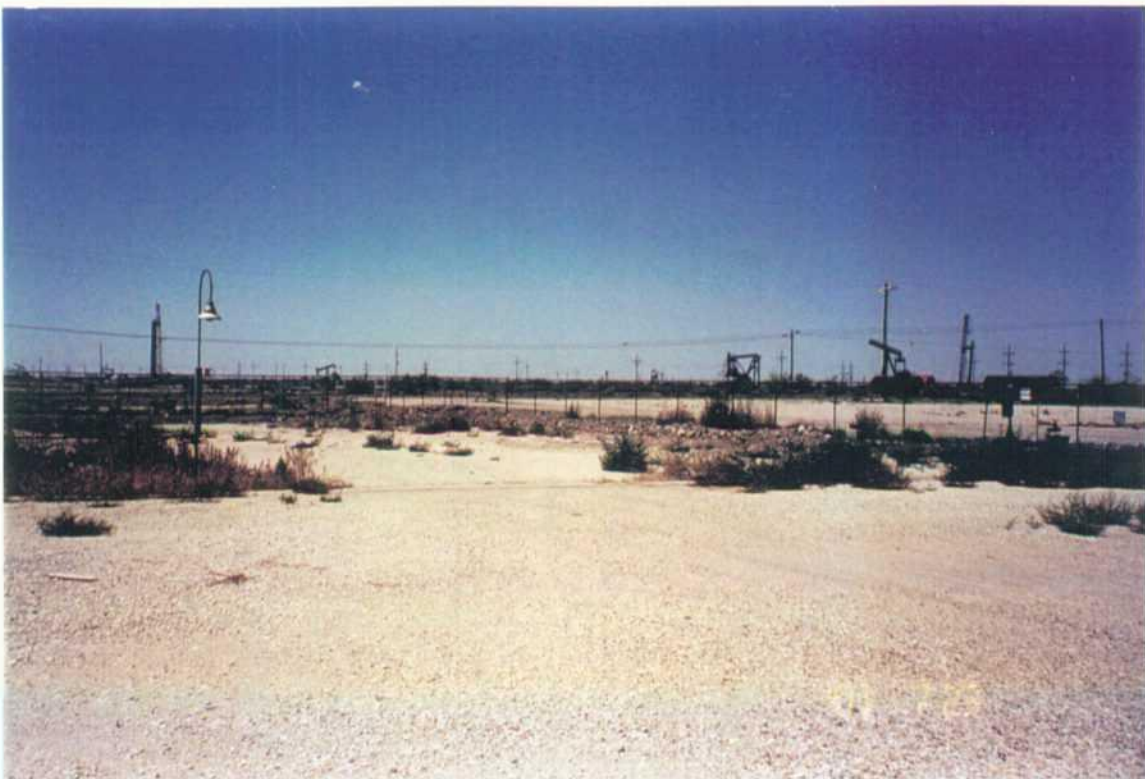
6. Storm Water Retention Berm (Looking Southwest)
