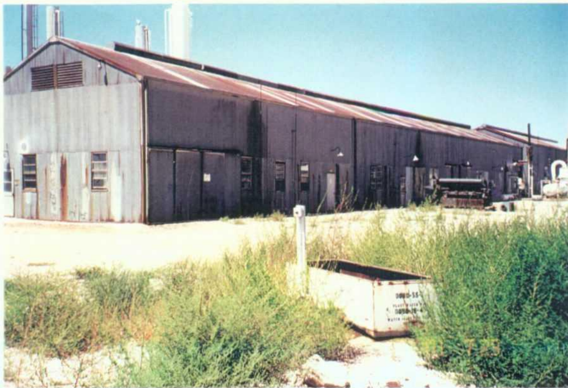
2. Plant Water Well
