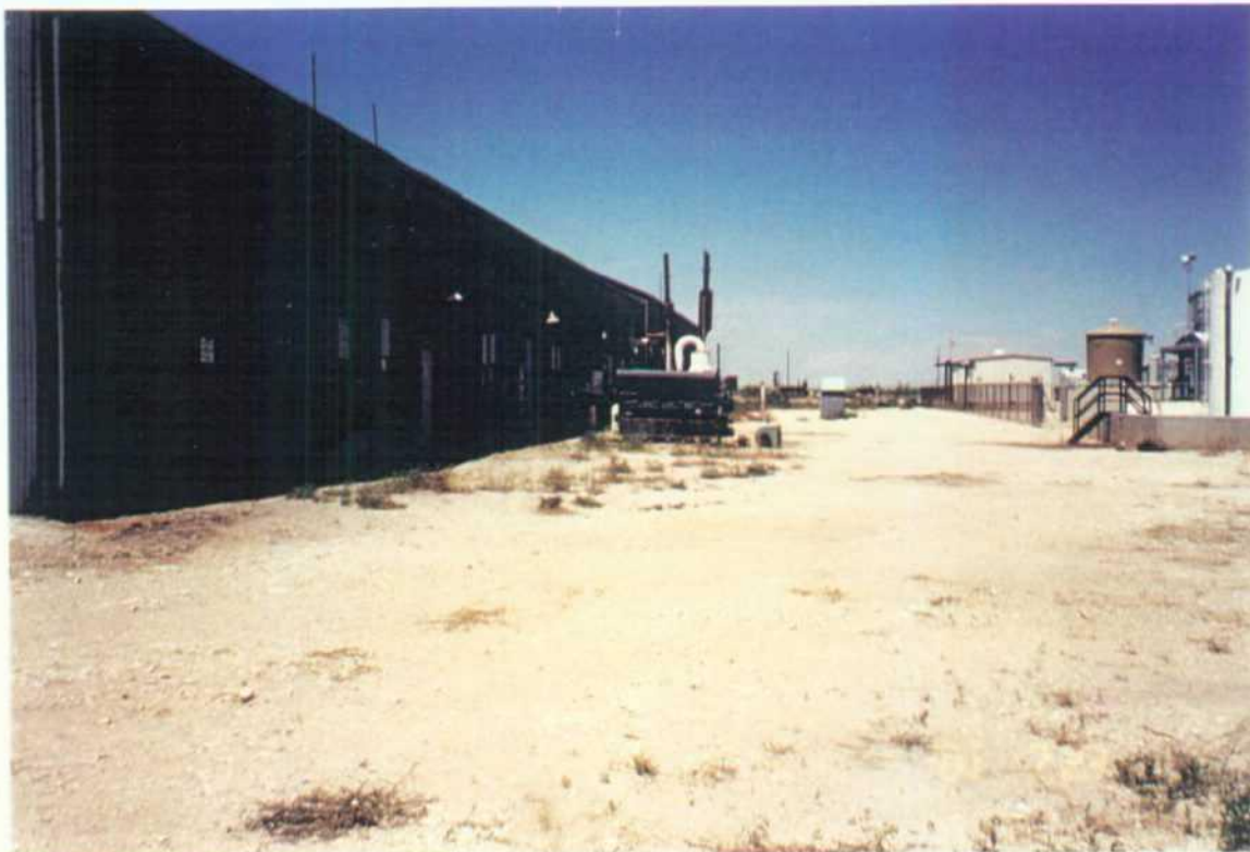
1. North Side of Compressor Building (Looking West)
