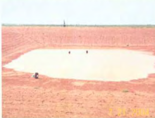
New clay lined pond-looking south- Infiltration devices in pond.
