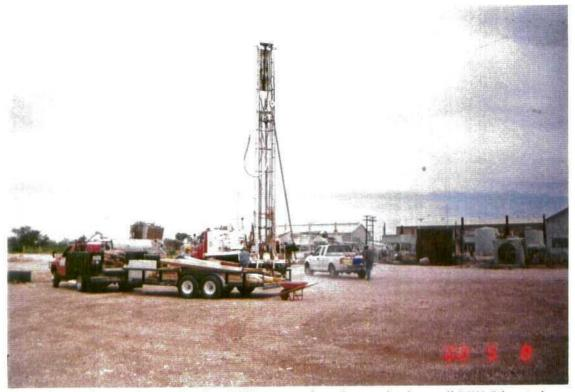
View facing northwest showing drilling operations for monitoring well MW-8 located approximately 180 feet upgradient (west) of monitoring well MW-4 and recovery well RW-1.
