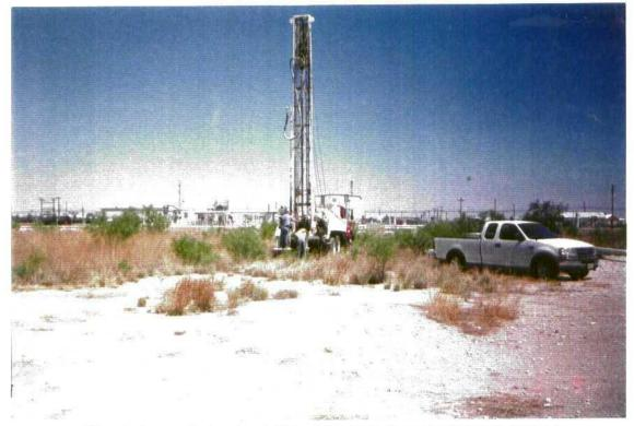
View facing north showing drilling operations at monitoring well MW-11 located approximately 650 feet downgradient (east) of monitoring well MW-1.
