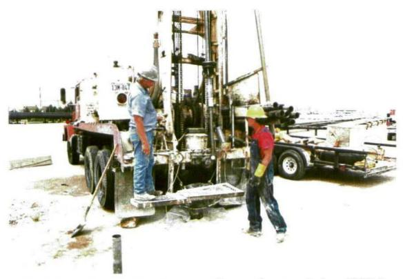
View facing northeast showing split-spoon sampling operations at monitoring well MW-5 located approximately 350 feet northwest of slop oil tank and 40 feet north of inlet gas scrubber.
