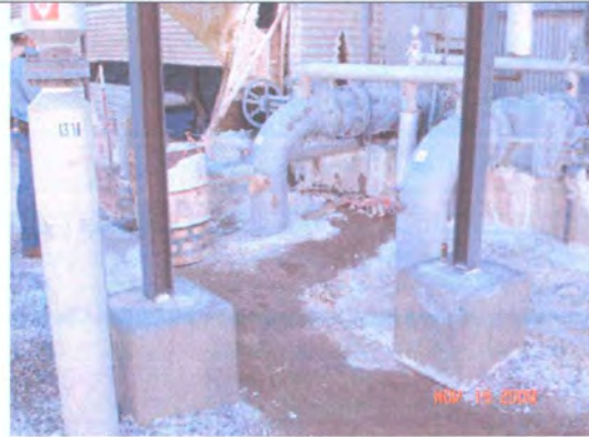
Photo 10: White residue near cooling tower.
