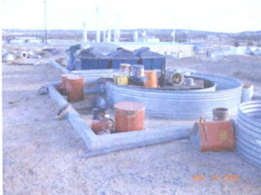
Photo 14: Containment for drained items.
