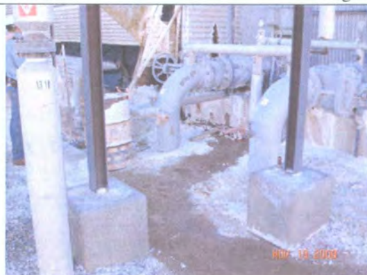
Photo 10: White residue near cooling tower.
