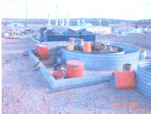
Photo 14: Containment for drained items.
