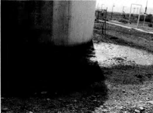
Photo 39: Discharges within earthen unlined bermed area from AST.
