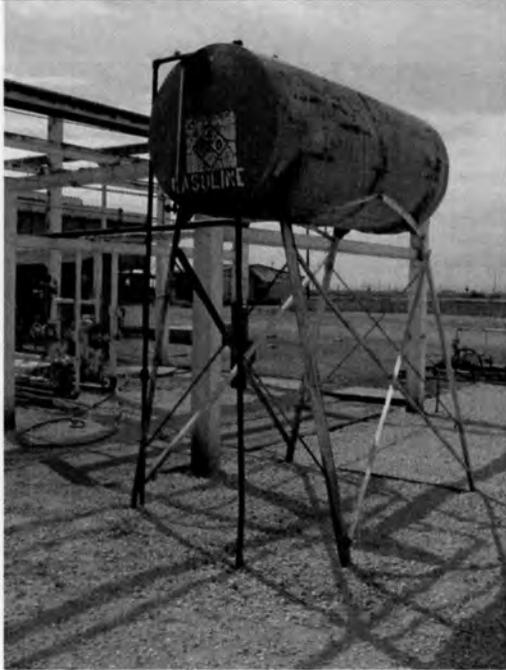
**Photo 37: Unbermed/lined saddle tank.**
