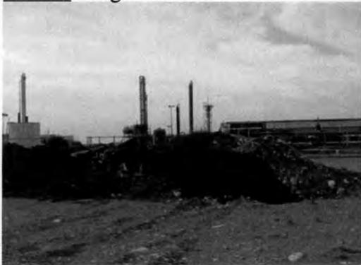
Photo 9: Staged contaminated soil.
