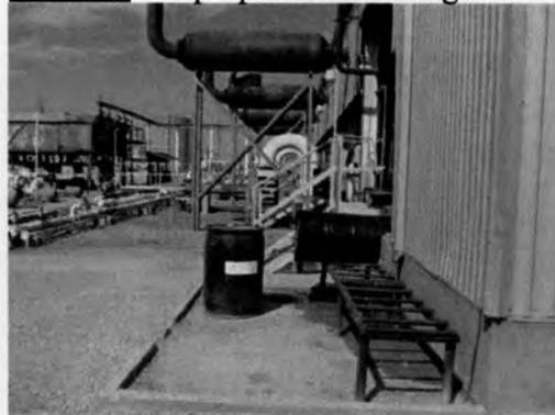
Photo 18: Improper barrel storage.
