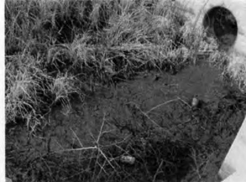
Photo 6: Old cooling tower containment full of black soil.
