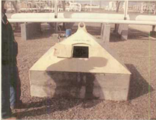
pyramid sump for used lube oil
