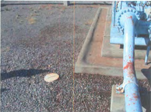
Photo 8: Hydrocarbon staining on the ground.
