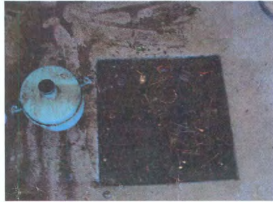
Photo 4: Sump being used as a below grade tank.
