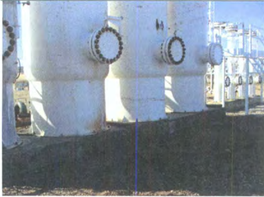
Photo 11: Arsenic treating unit has discharge on ground.
