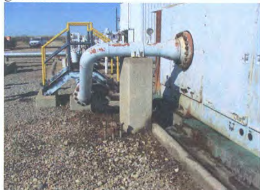
Photo 10: Hydrocarbon staining on the ground.
