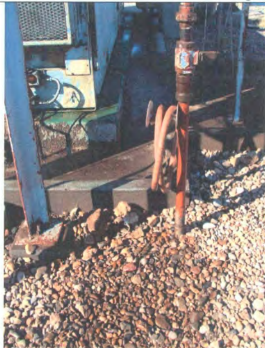
Photo 9: Hydrocarbon staining on the ground.
