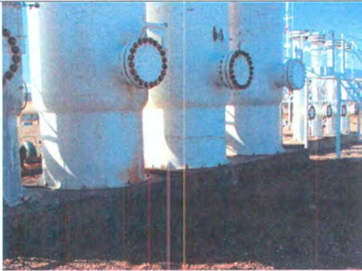
Photo 11: Arsenic treating unit has discharge on ground.
