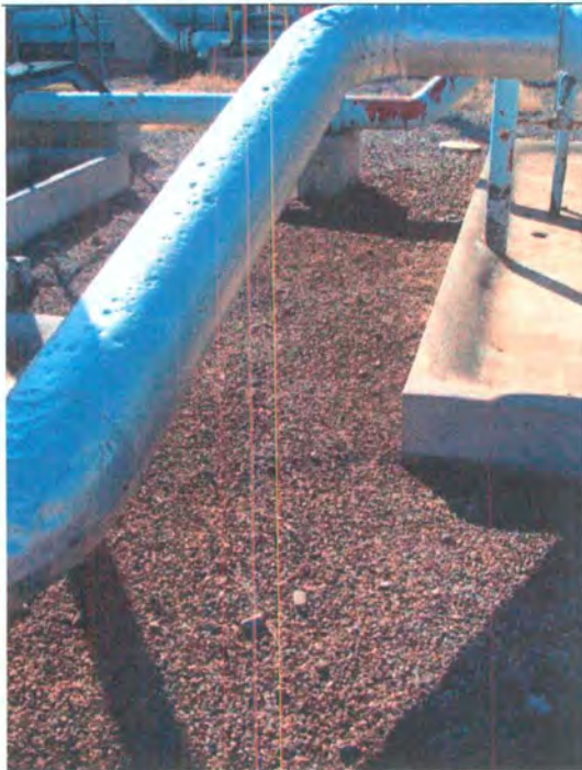
Photo 7: Hydrocarbon staining on the ground.
