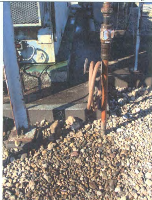
Photo 9: Hydrocarbon staining on the ground.
