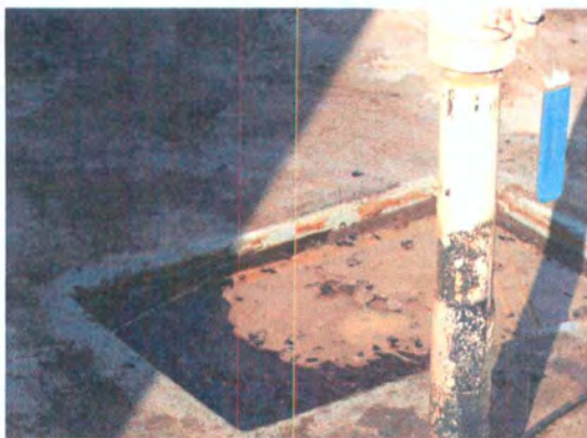
Photo 1: Sump being used as a below grade tank.
