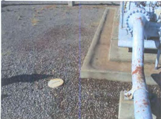
Photo 8: Hydrocarbon staining on the ground.
