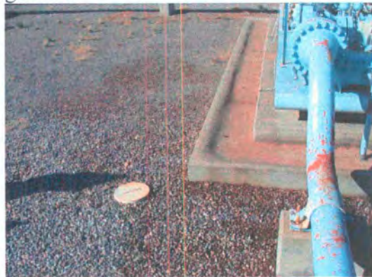
Photo 8: Hydrocarbon staining on the ground.
