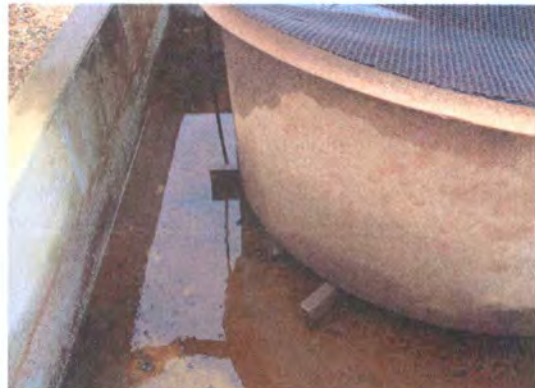
Photo 6: Standing fluids in a secondary containment.
