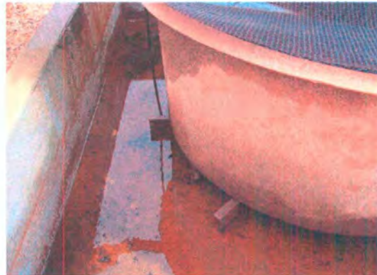
Photo 6: Standing fluids in a secondary containment.
