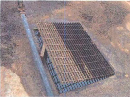
Photo 2: Sump in secondary containment used as a below grade tank.
