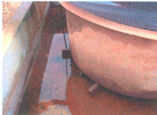
Photo 6: Standing fluids in a secondary containment.
