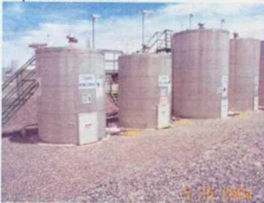
Tank Farm. Tanks have concrete pads under each tank. They are setting on a compacted area.
