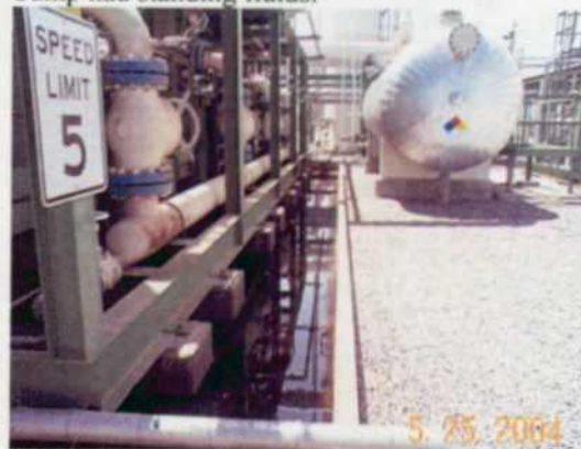
Another process unit. Process unit with Amine and water standing in the pad and curb area.
