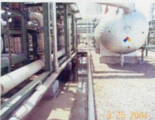
Process units with Amine and water standing in the pad and curb area.
