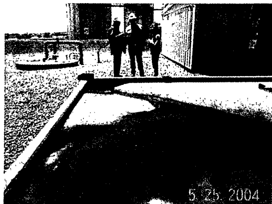
Steam and wash off pad with single line sump. Sump had standing fluids.
