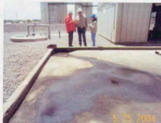
Steam and wash off pad with single line sump. Sump had standing fluids.
