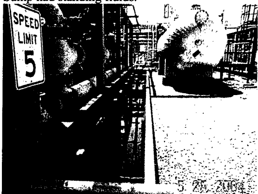
Another process unit. Process unit with Amine and water standing in the pad and curb area.
