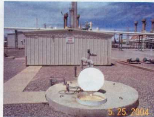
One of two main below grade tanks with secondary containment.
