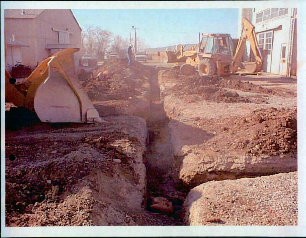
NEW DRAIN LINE PITCH. RUNNING EAST & WEST. LOCATED SOUTH OF & 6 BOILER
