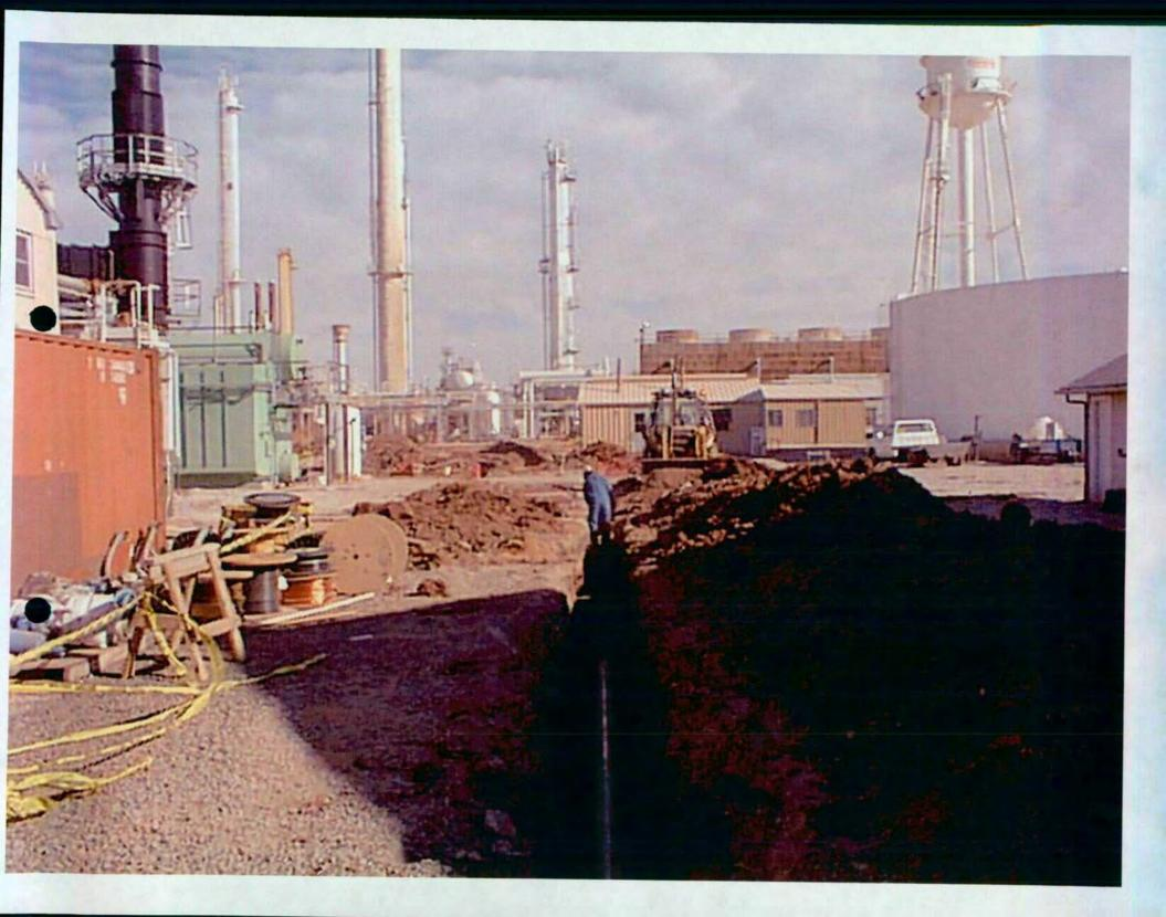
NEW 6" DRAID LINE RUNNING EAST 4WEST SOUTH OF "6 BOILER
