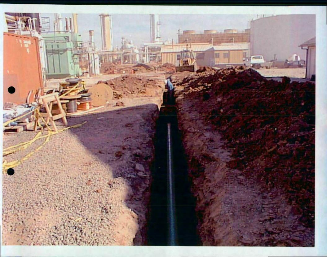
NEW DRAIN LINE MAIN LINE 6" CONTER PIPE
